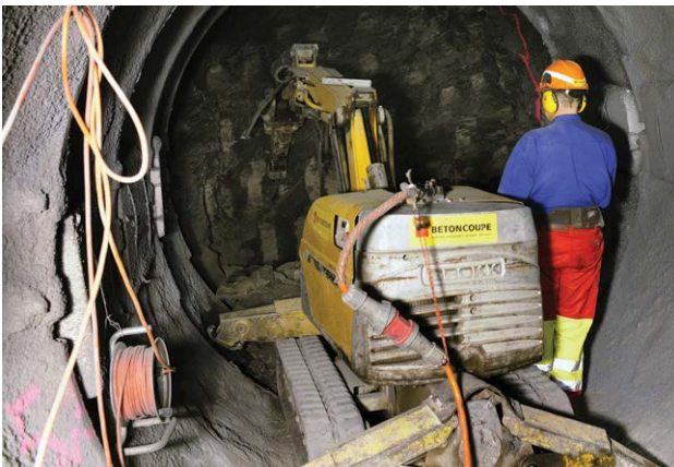
Excavation of a drift in Opalinus Clay for the Full Scale Emplacement Experiment (Mont Terri Underground Rock Laboratory, Switzerland) (© Comet Photoshopping).
