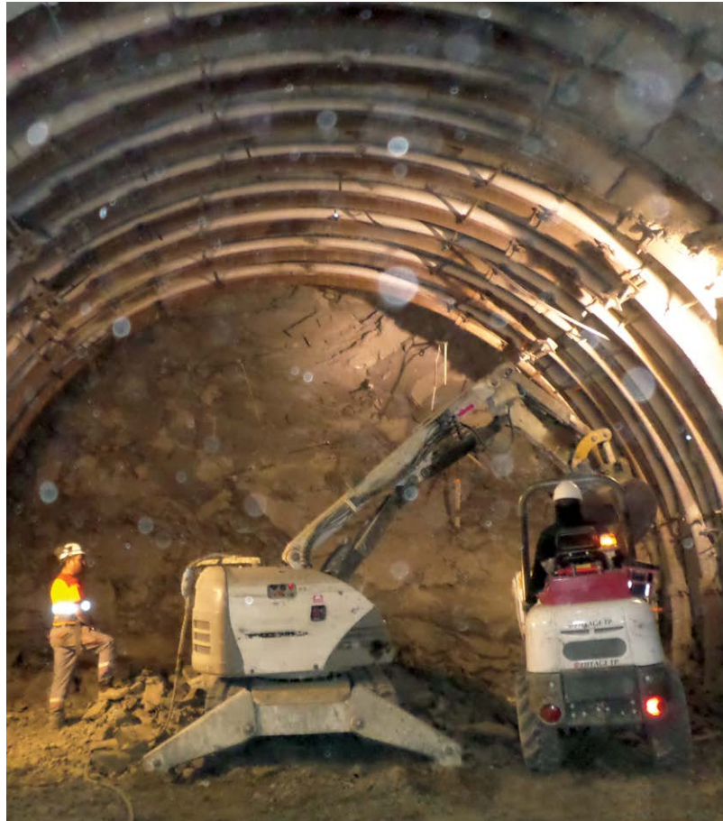
Excavation of a drift in Callovo-Oxfordian clay (Bure, France) (source: Andra).
