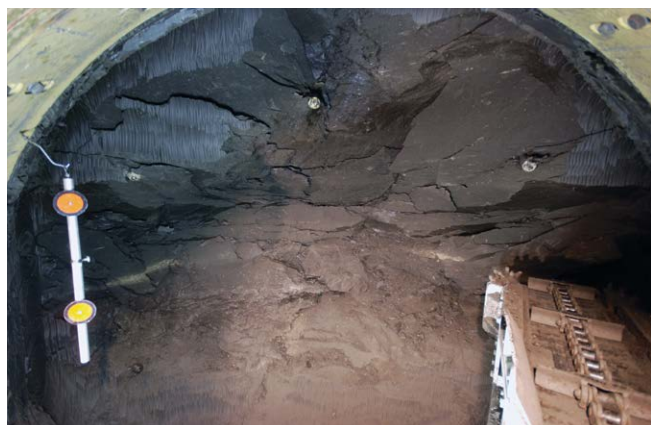
Construction of a shaft (left) and excavation of a drift (right) in Boom Clay (Belgium) (source: EURIDICE).
