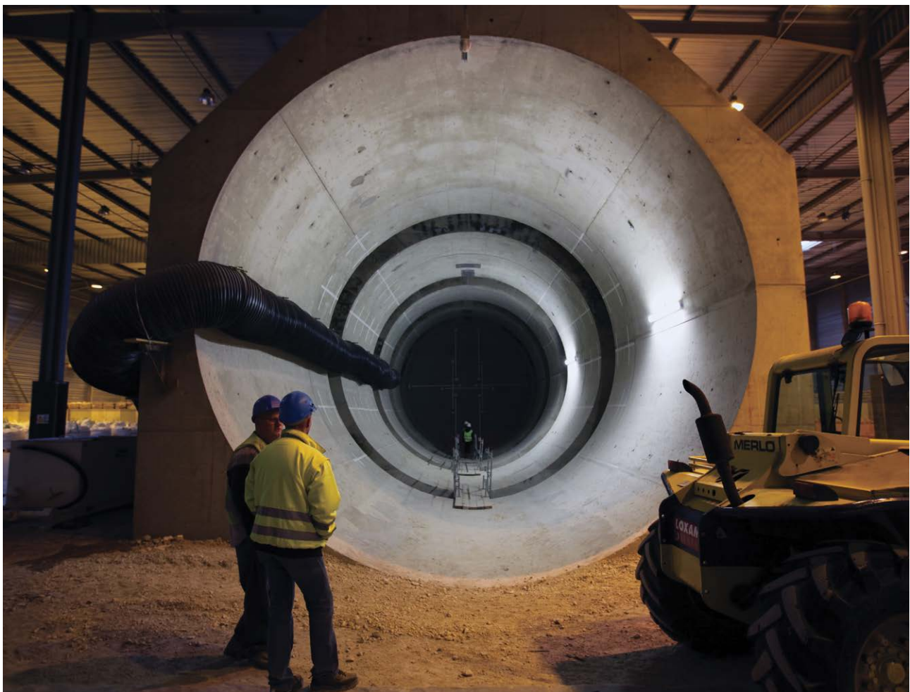
Figure 10 – Full-scale seal experiment (France). This experiment is a technological demonstration performed above surface by Andra with the scientific support of Nagra, within the DOPAS European project. The test box is 36.1 meters long, with an inside diameter of 7.6 meters. A seal has been installed inside the test box (after the picture was taken), according to the sealing concept presented in Figure 9. The containment plugs are 5 meters long and the swelling clay core is 13.5 meters long (B.TINOCO©Andra).
