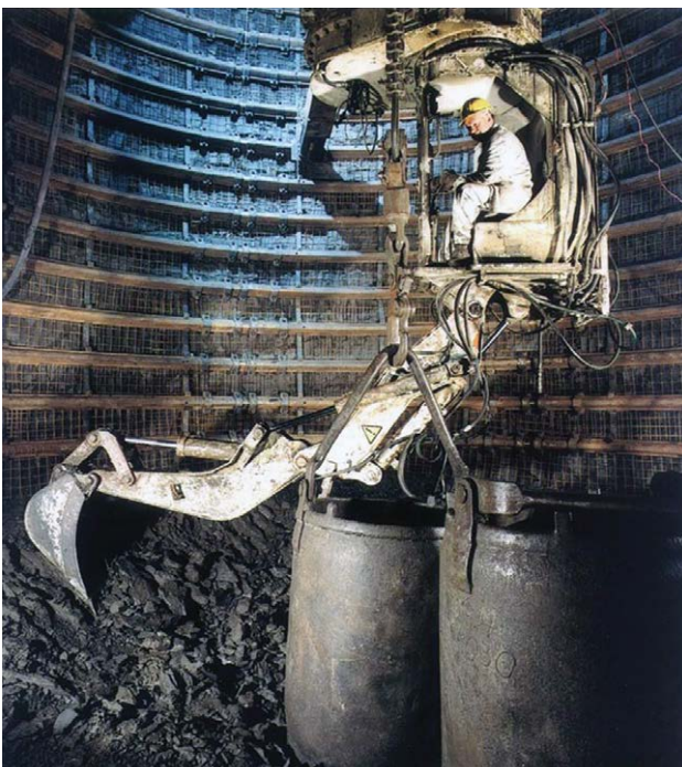
Construction of a shaft (left) and excavation of a drift (right) in Boom Clay (Belgium) (source: EURIDICE).
